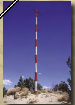
The candy-striped homing pole in the White Sands Play Area serves as a visual reference point. A beacon light is on at night.
